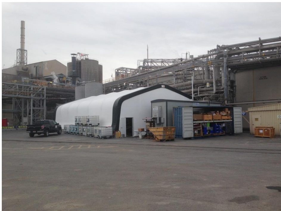
Figure 1: The Demonstration Plant on site
